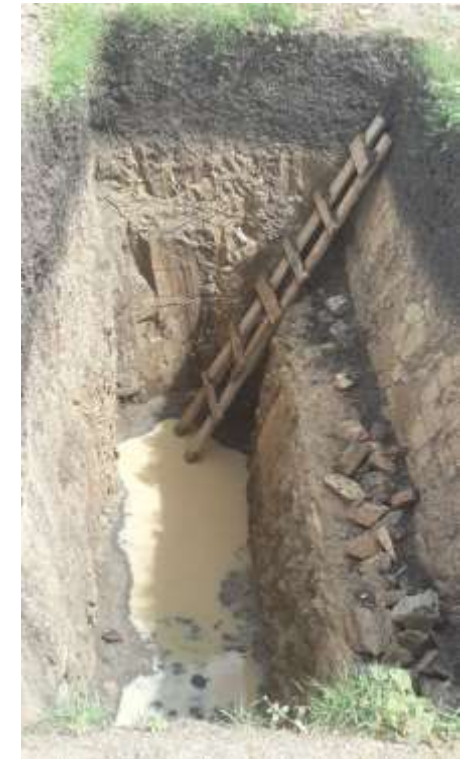
Loose soils, often water logged and rocky grounds- Lodoi Primary School- 8/12/2014
