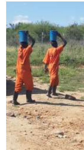
Females providing water for curing blocks- Katikit P/S- Dec 2014
