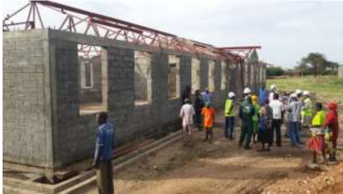
PMP Site inspection including community members- Lotome P/S- December 2014
