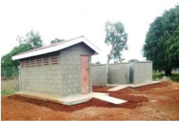
6 Stance V.I.P Latrine and Shower Block - Orwamuge P/S- April 2015
